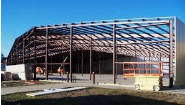
Erection of a pre-engineered metal building
