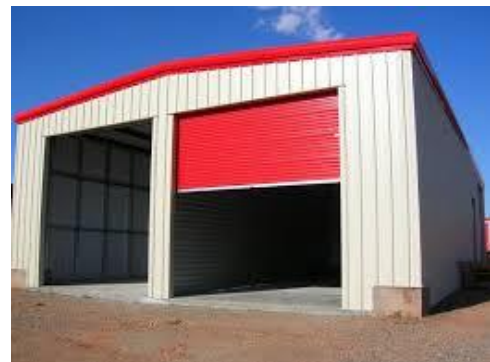
A completed pre-engineered metal building
